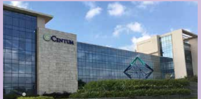
Facility in Bangalore Aerospace Park
