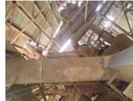
Replacement of CR Elevator discharge chute in SSP Plant
