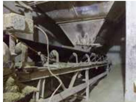
Replacement of RM Feed Belt in PSSP Plant
