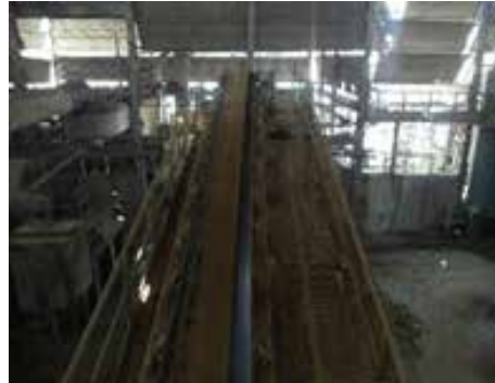
Replacement of Production belt in PSSP Plant
