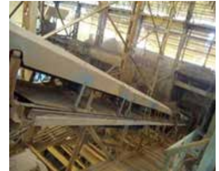
Installation of canopy over inclined Conveyor belt in SSP Plant
