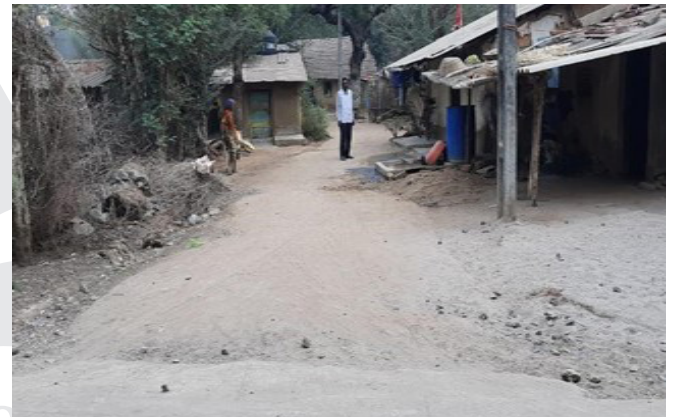
After Construction of Soakpit
