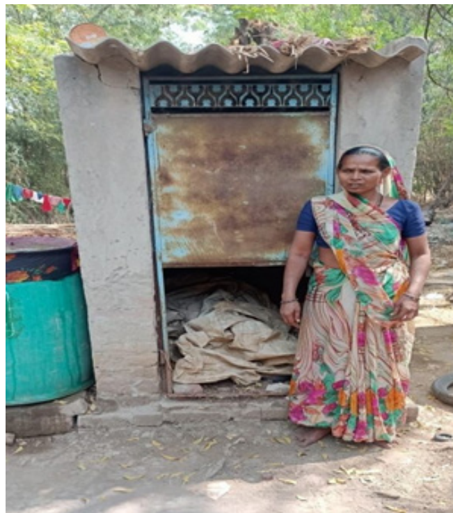
Earlier Toilet used as storeroom
