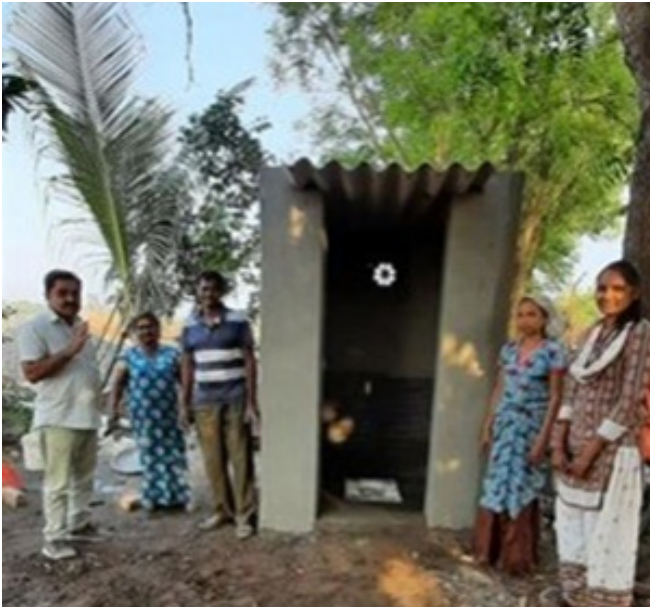
Newly Constructed Toilets
