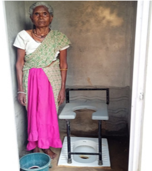
Newly Constructed Toilets with Facilities for Elderly
