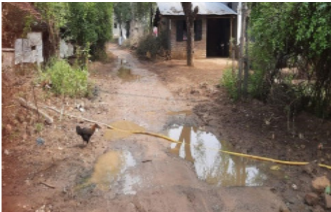
Before Construction of Soakpit
