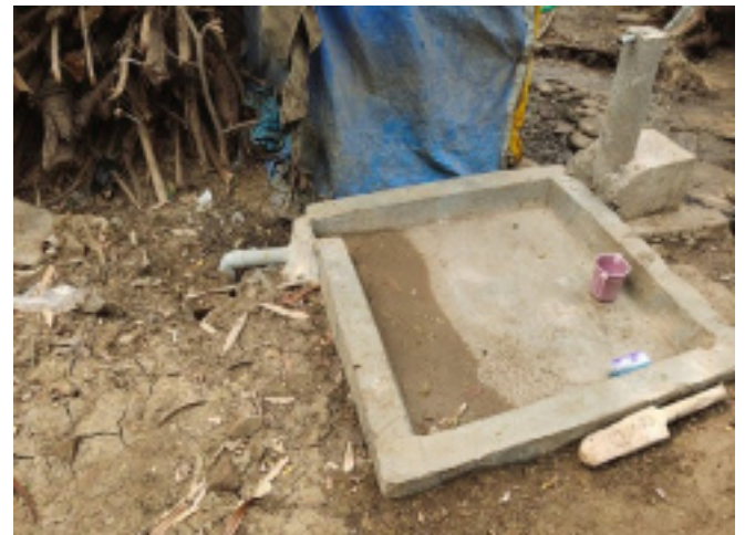
After Construction of Washing Platform
