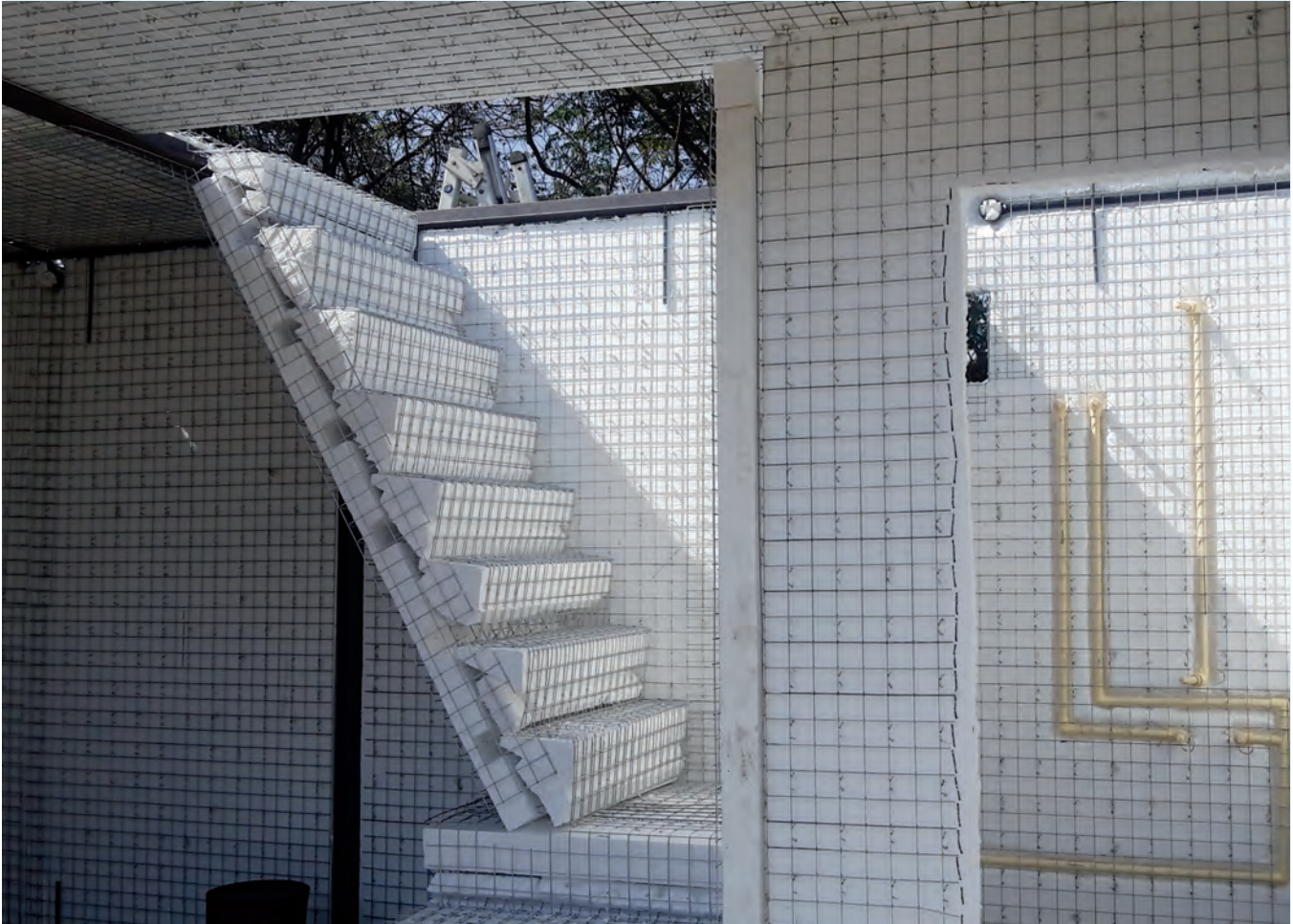
The making of the house – putting in electrical & plumbing lines.
