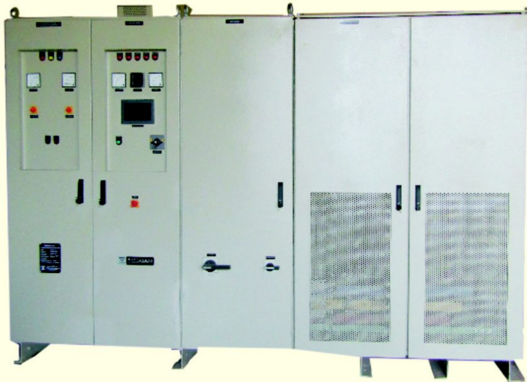
SUPPLY OF 200V / 3200A SCR CONTROLLED (12 PULSE) RECTIFIER TO BGR ENERGY SYSTEMS FOR ELECTRO CHLORINATION PROCESS
