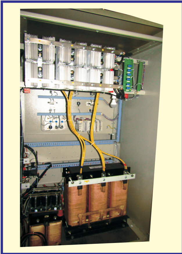
SUPPLY OF 100V / 150A DC RECTIFIER TO POWER PLANT FOR CATHODIC PROTECTION
