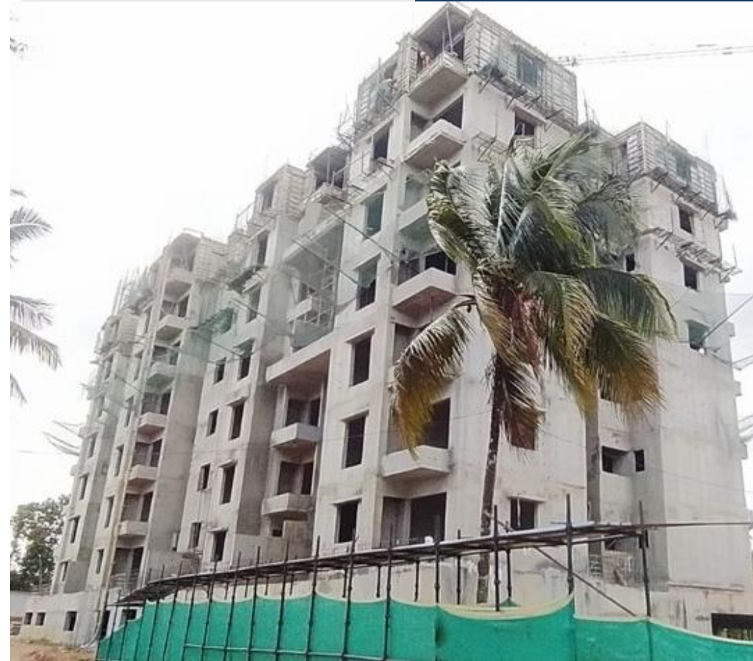
Tower A - 8th Floor Slab WIP
