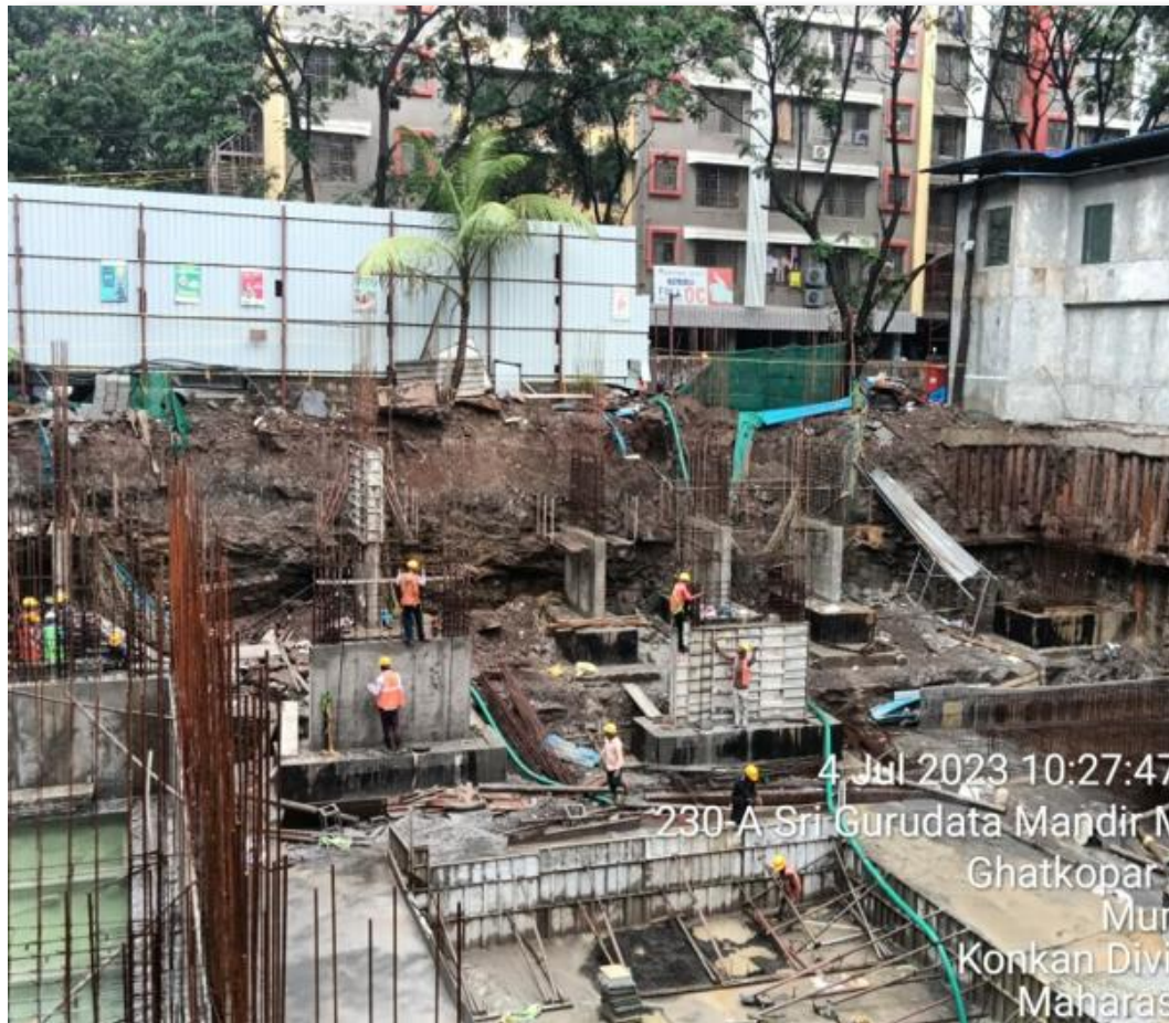
Column Work - Open Footing WIP
