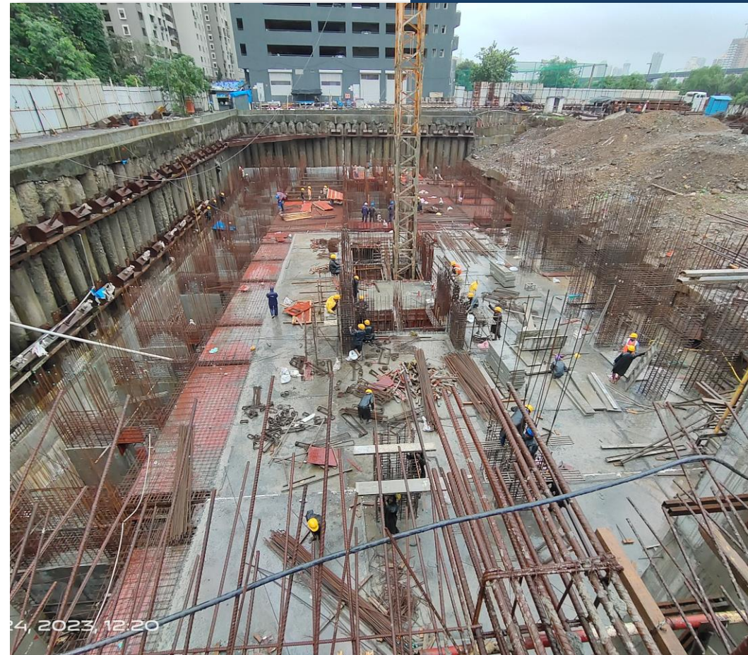
Tower A B-2 Slab Decking WIP
