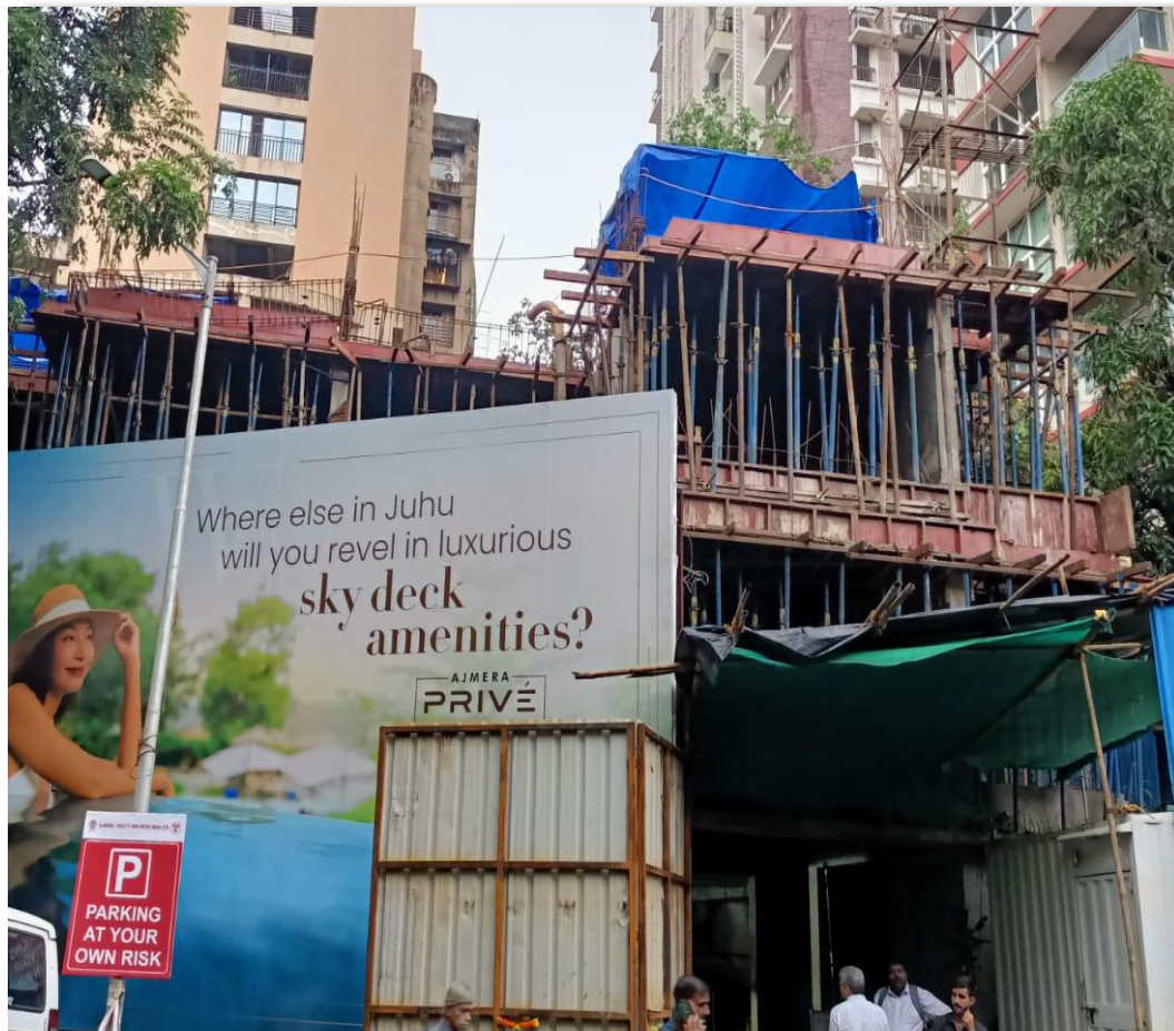
2nd Floor Slab Casted
