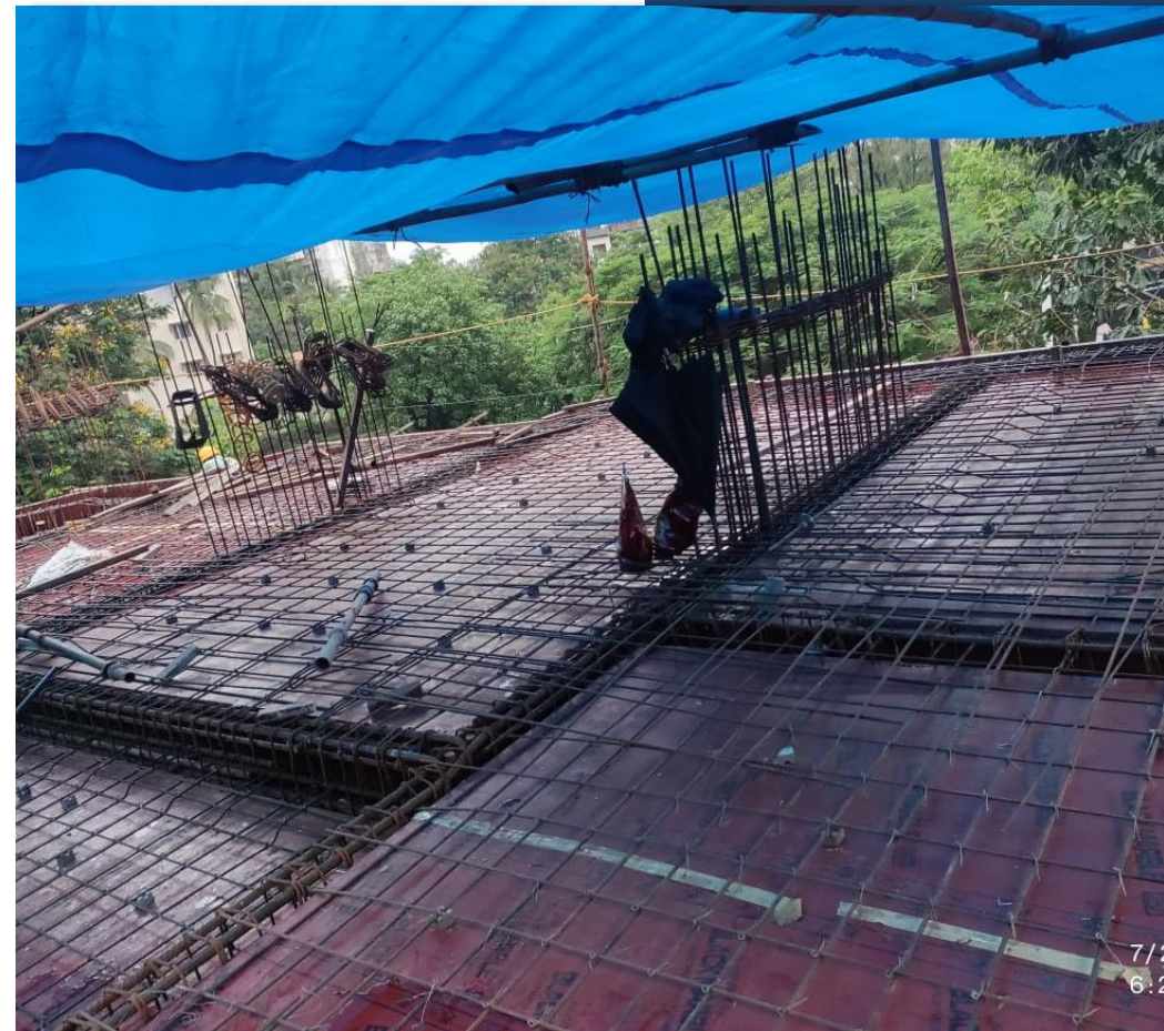
Reinforcement Work for 3rd Floor Slab
