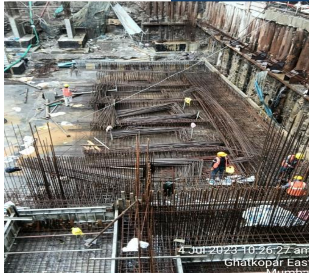
Raft Reinforcement WIP
