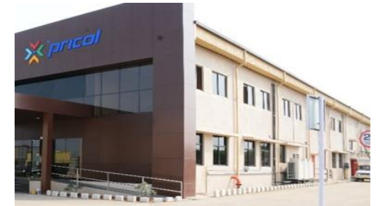
Plant - 5 Pune, Maharashtra
