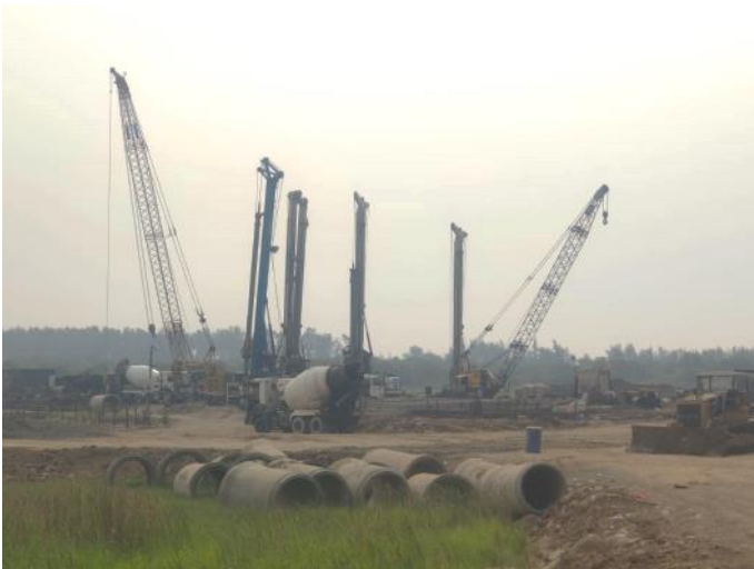
Exhibit 11: Excavation in progress at SBR Vasai
