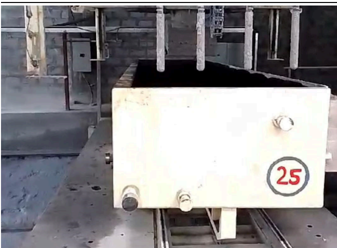
Fig 5 – AAC slurry is collected in an oiled mould and cooled to form a cake
