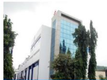
API Plant III - Patalganga
